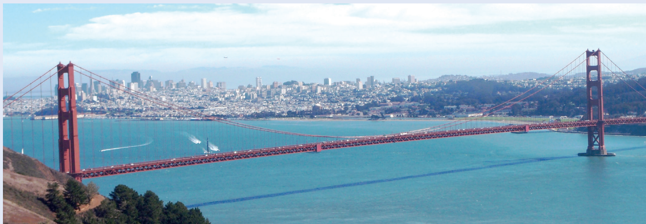
Golden Gate bridge.
